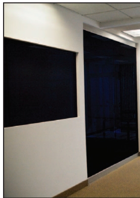
SPD-SmartGlass in the dark and clear states at the Research Frontiers Design Center
